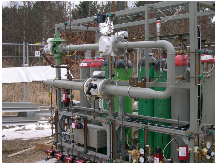
Figure 4: The actual construction of the test cycle for the industrial gas flowmeters. The compressor is situated in the grey box at the left bottom of the picture.
